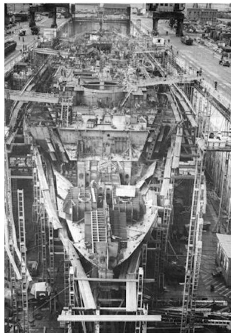
Construction of *USS Kentucky* in 1946. Construction intermittently continued until she was about 75% complete. The *Kentucky* was never completed, and she was scrapped in 1958. Her machinery was carefully removed and used to power two fast Combat Support Ships - the *USS Sacramento* (AOE1) and *USS Camden* (AOE 2). (Iowa Class BB's / Sumrall)
