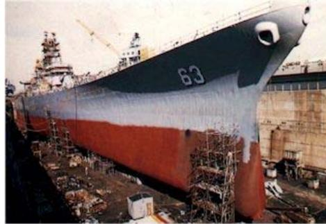
The USS Missouri under construction. Her sleek external lines provide no evidence of the massive armor belts that lie underneath.
